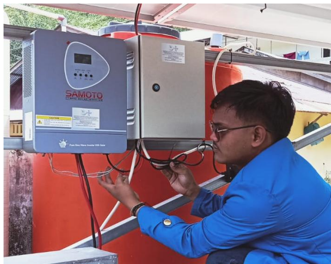
Gambar 4. 3 Instalasi Inverter Hybrid
