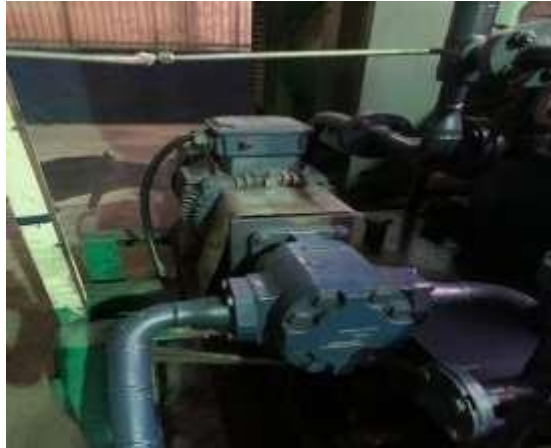
Gambar 2.10 Electrical Oil Pump (PT. Adibrata Unggul Jaya)
