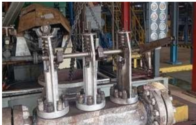
Gambar 2.9 Spindle Valve (PT. Adibrata Unggul Jaya)
