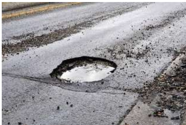
Gambar 2.19: Lubang ( Potholes )
