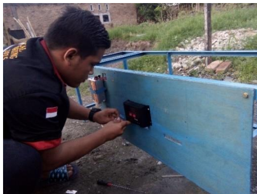
Gambar 3.32 Memasang Charger Controller
