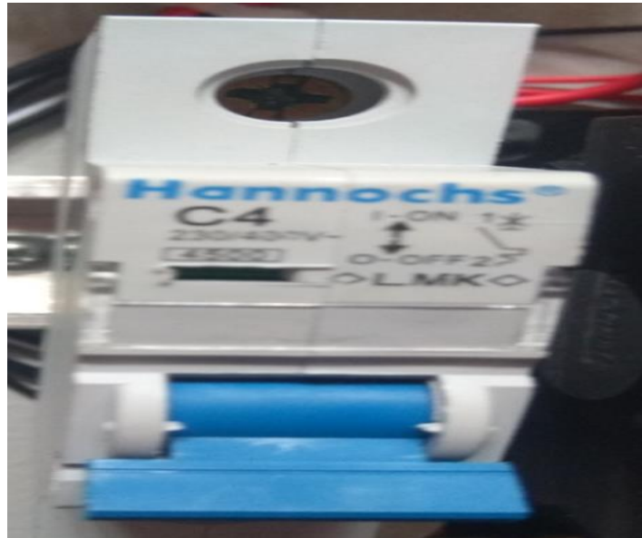
Gambar 3.7. MCB (Miniature circuit breaker)
