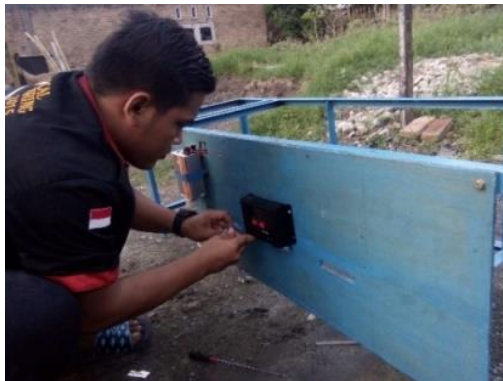
Gambar 3.27 Memasang Charger Controller
