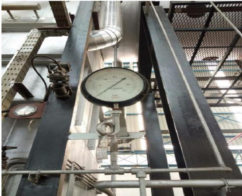
Gambar 3.10 Pressure Gauge Ketel Uap
