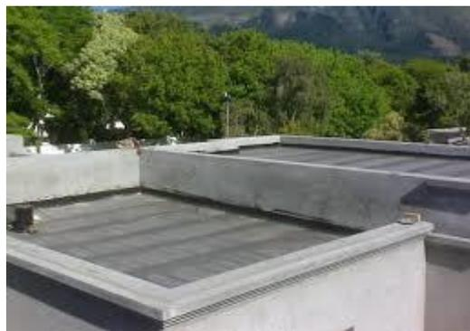
Gambar 2.6 Atap Dak Beton
