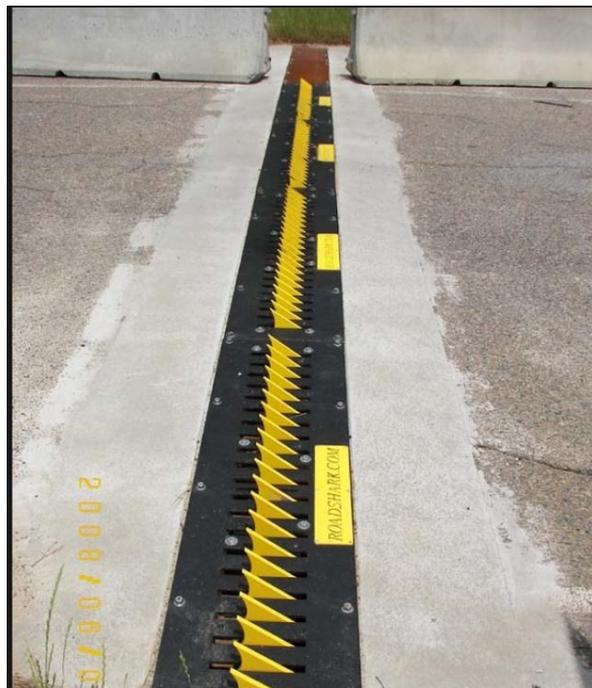
Gambar 2.5 *Flush-mounted Traffic spikes* (Roadshark International inc, 2016)
