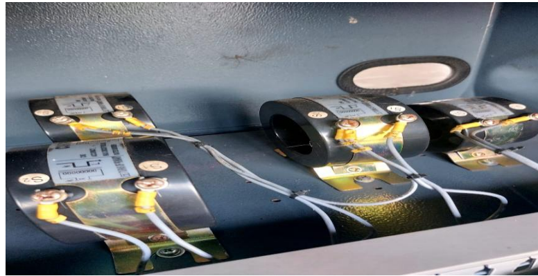
Gambar 2.2.17 Cylinder Current Transformer (CT)
