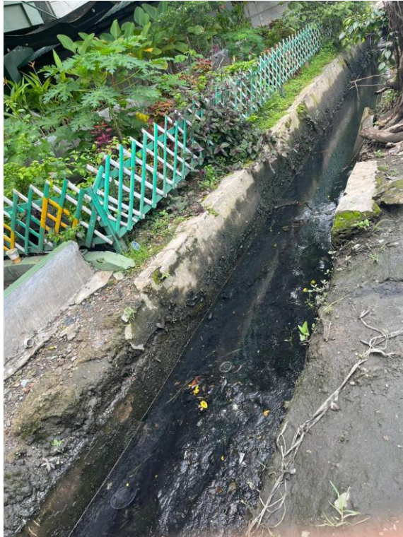
Lampiran 5. Survey Drainase Sekunder 3 Lokasi Peneletian
