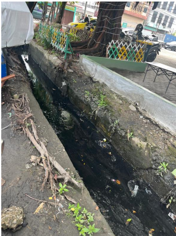
Lampiran 4. Survey Drainase Sekunder 2 Lokasi Peneletian
