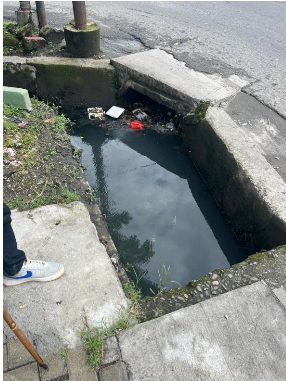
Lampiran 3. Survey Drainase Sekunder 2 Lokasi Peneletian
