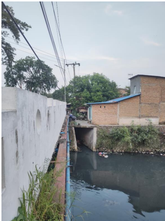
Lampiran 6. Survey Drainase Sekunder 3 Lokasi Peneletian
