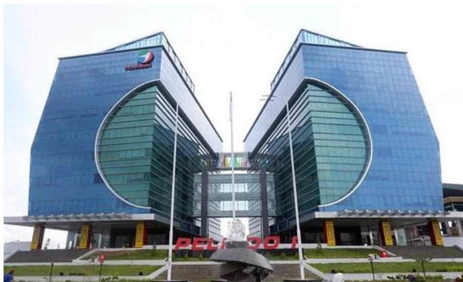
Gambar 4.1 Kantor Pelindo Multi Terminal
