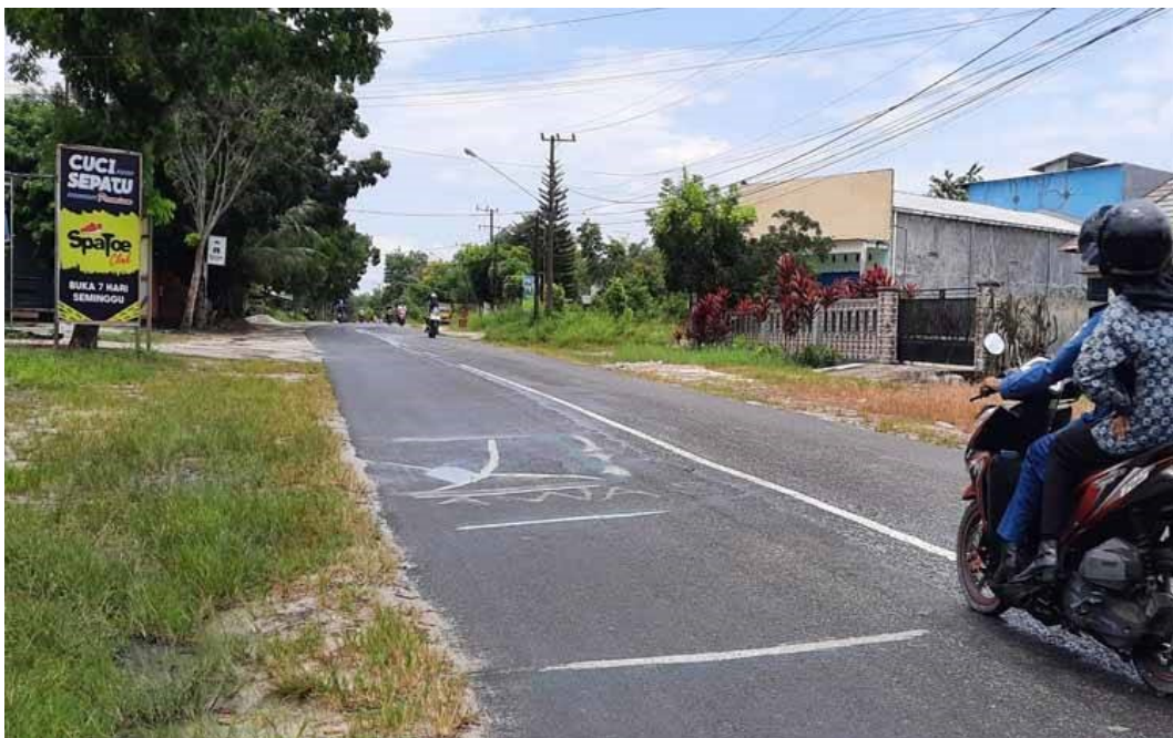
Gambar 2.4: Cekungan ( Bump and Sags )
