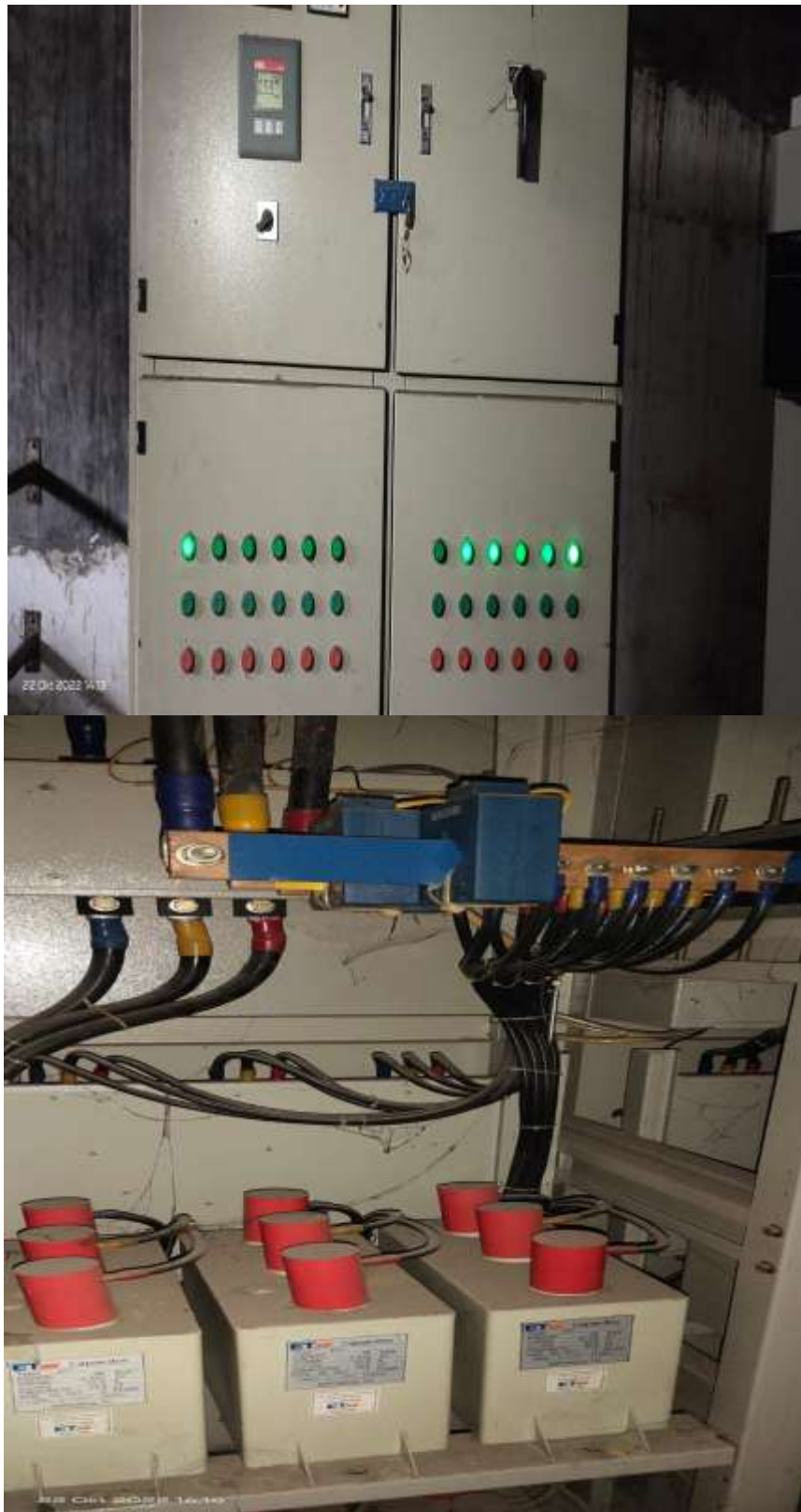
Gambar 4.2 Panel Kapasitor Bank
