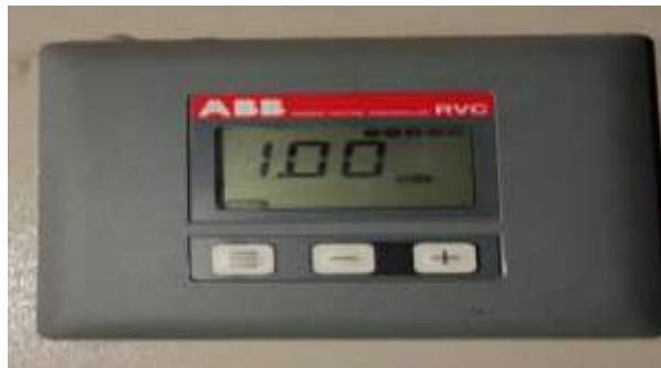
Gambar 4.3 Power Factor Controller (ABB)
