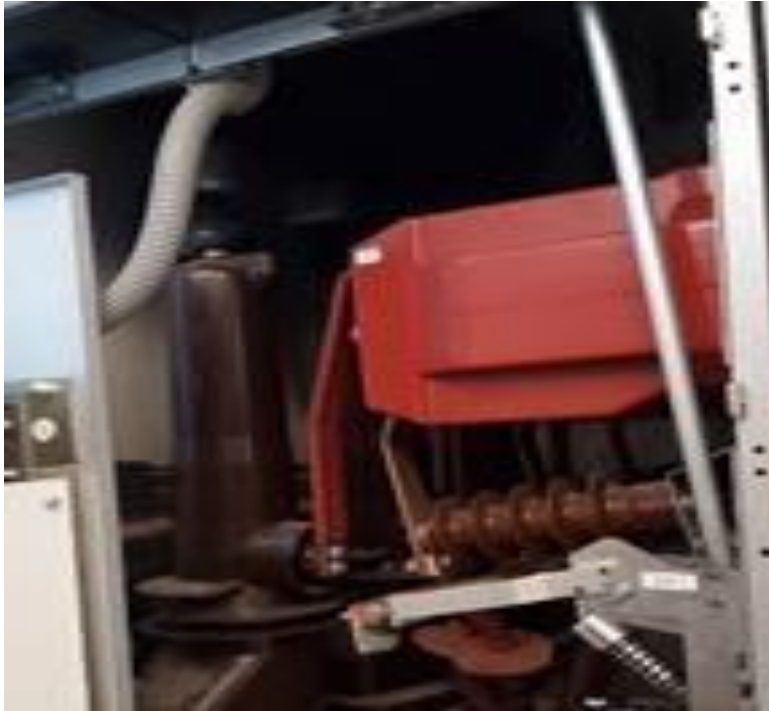
Gambar 2.10 Current Transformator (CT)
