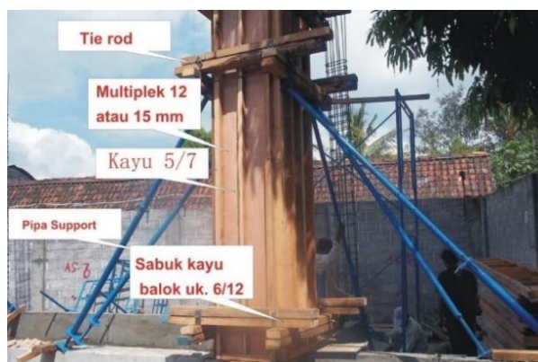
Gambar 2.1 : Bekisting konvensional (Nugroho, 2018)
