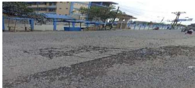
Gambar 3. 5: *spalling corner* (survey lokasi)
