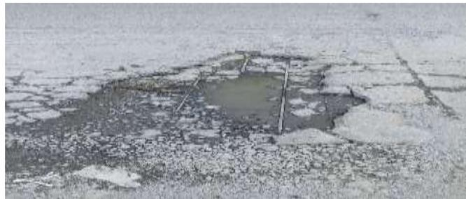
Gambar 3. 4: *spalling joint* (survey lokasi)
