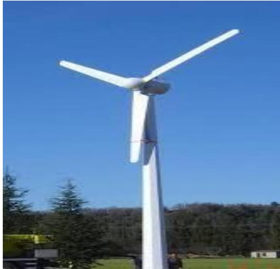
Gambar 2.1 Turbin Angin Sumbu *Horizontal*
