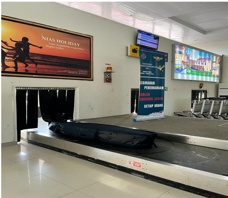
Gambar L.12 Baggage conveyor belt
