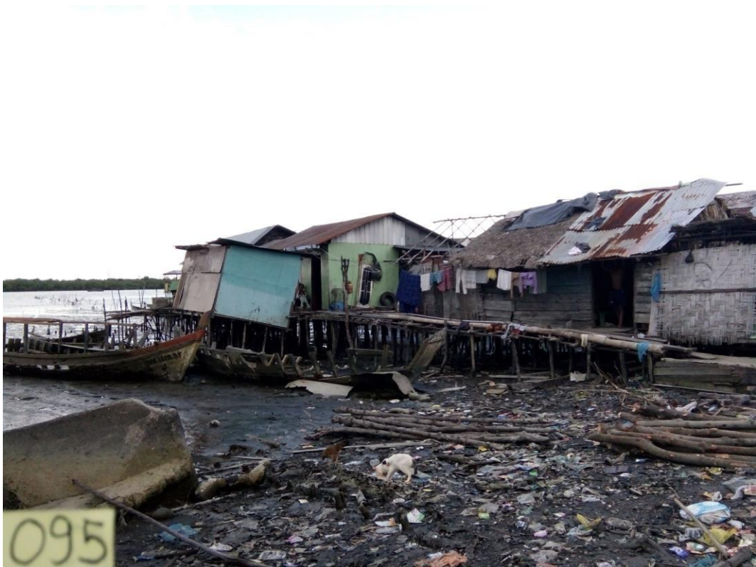
Lampiran 1. 6 Kondisi Marking 095
