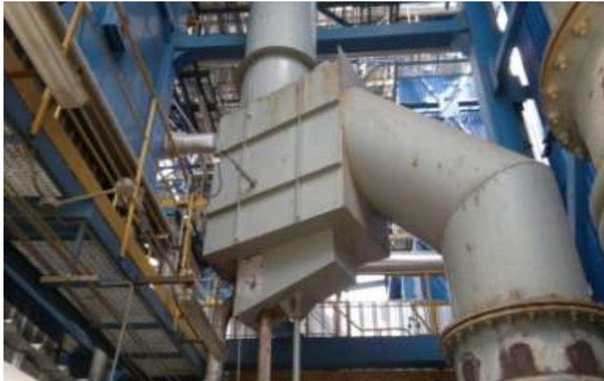
Gambar 2.10 Loop Seal
