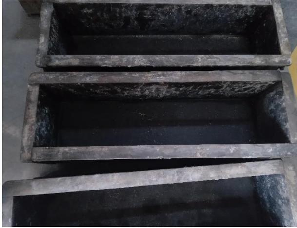
Gambar L-25: Bekisting balok.
