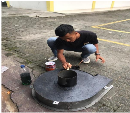
Gambar 4.29 Proses Flinkote
