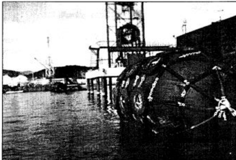
Gambar 2.22: Fender pneumatic (Triatmodjo, 1996)
