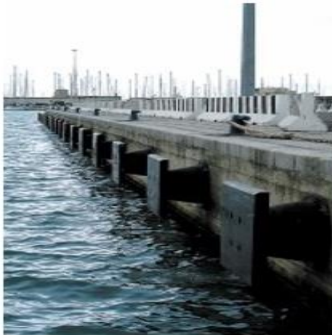
Gambar 2.23: fender super cone (Fentek marine fendering system)
