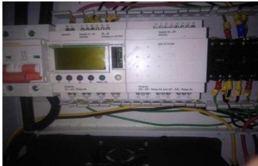
Gambar 2.1 Smart Relay SR3B101BD Schneider .
