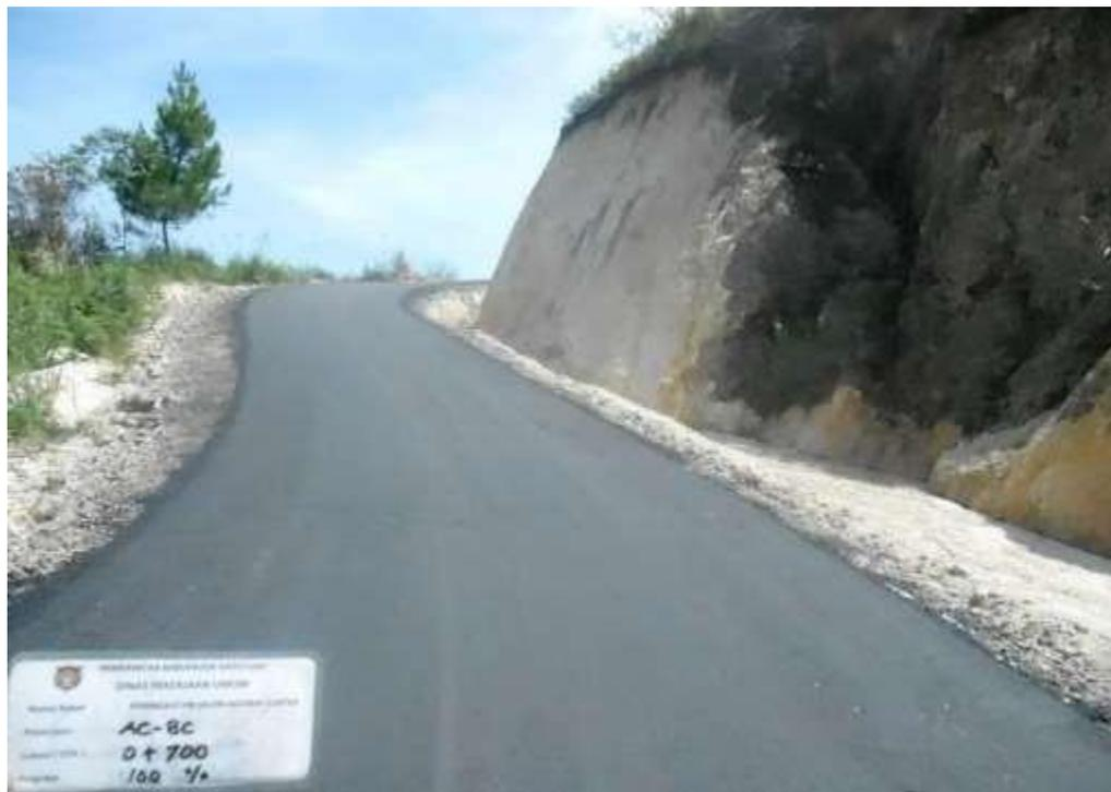
Gambar L8: Lapisan perkerasan AC-BC
