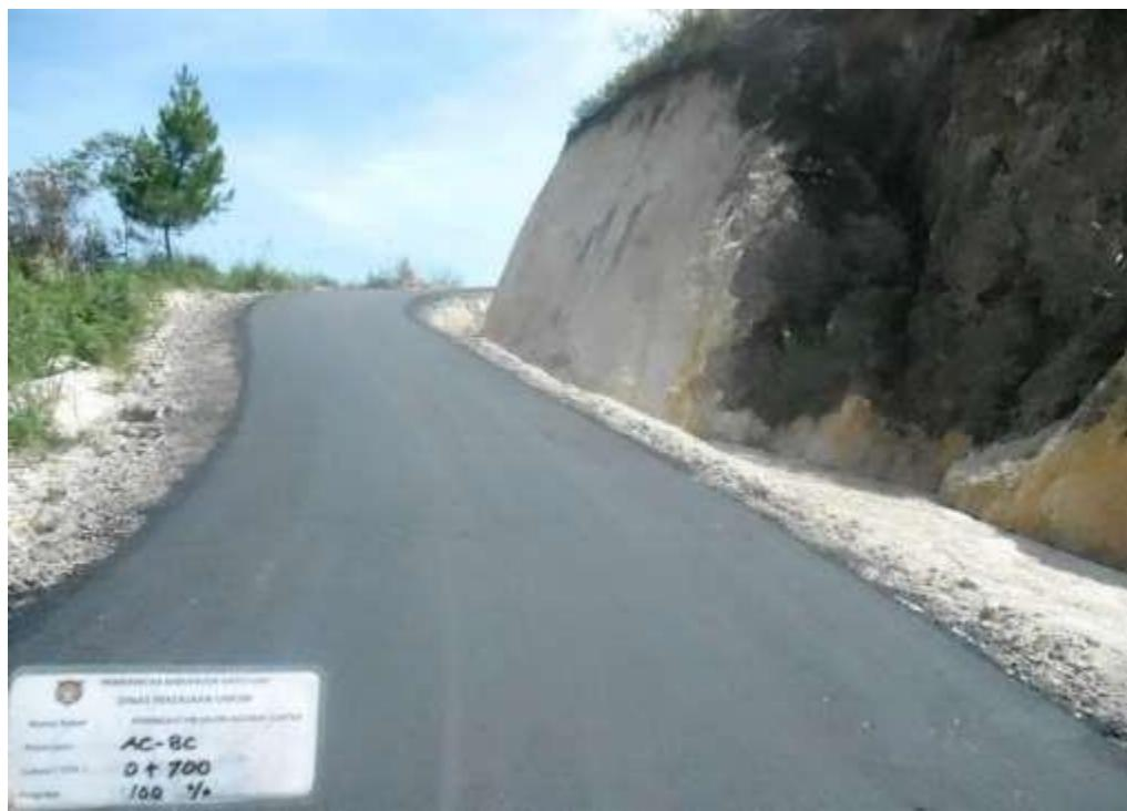
Gambar L8: Lapisan perkerasan AC-BC
