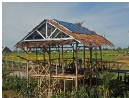
Gambar 4.1 Posisi Panel Surya
