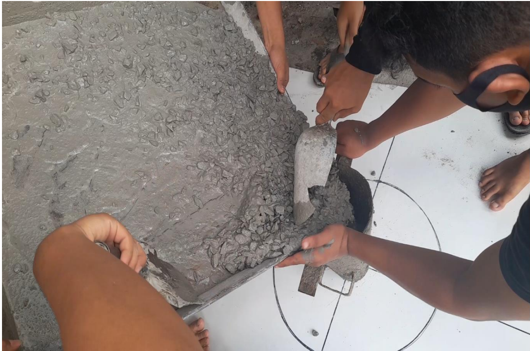
Gambar L.19: Proses Pengujian Slump Flow .
