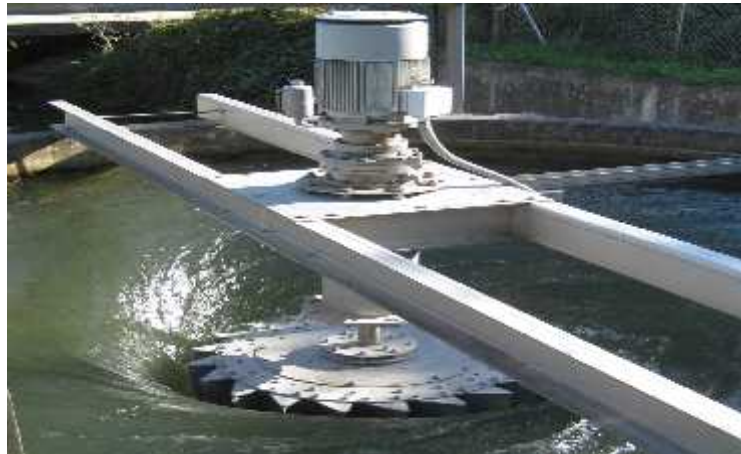
Gambar 2.6 Turbin Vortex
