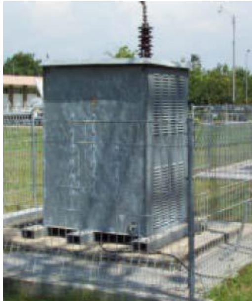
Gambar 2.11 Neutral grounding resistance (NGR)
