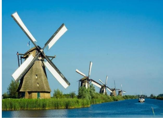
Gambar 2.4 turbin angin tipe *Dutch Four Arm*
