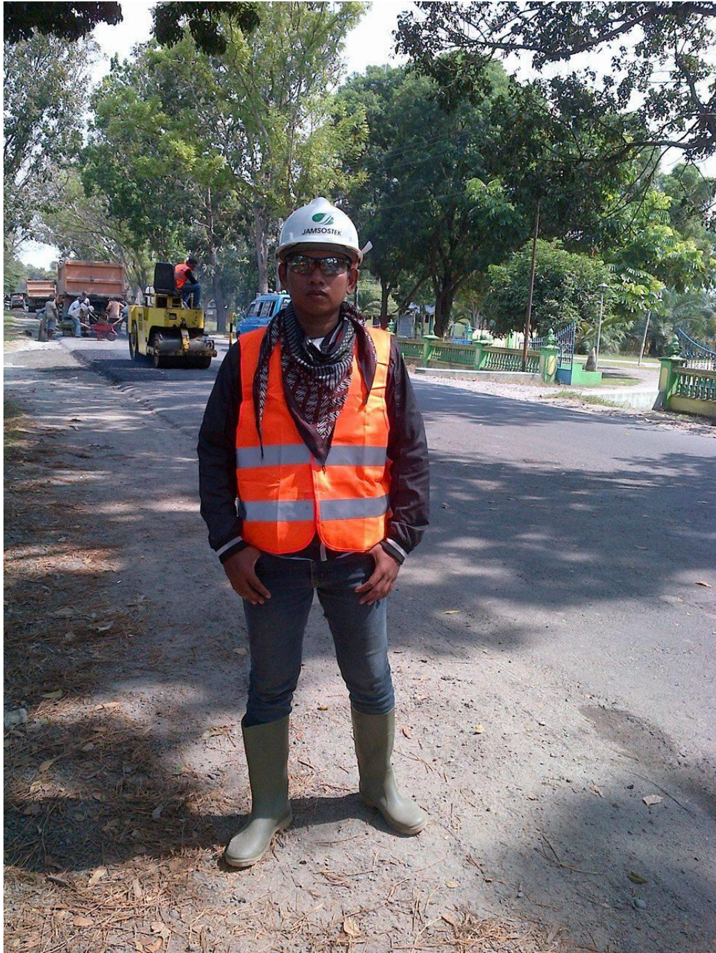
Gambar L3: Kondisi saat pelaksanaan Penambalan ( Patching )
