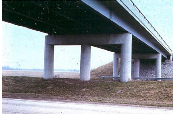
Gambar 2.1: Multi-Column Pier di jalur antar kota ( https://www.dot.state.oh.us ).
