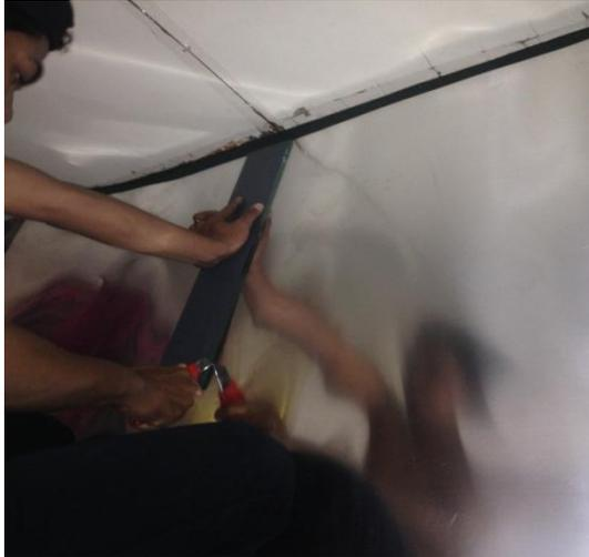
Gambar 3.20 Memotong Plat Aluminium
