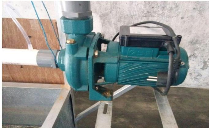
Gambar 3.3. Pompa Sentrifugal
