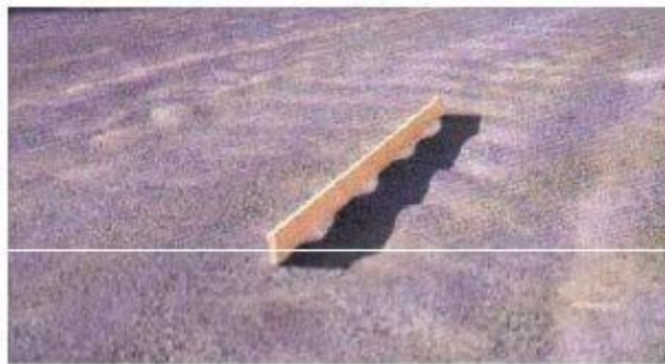
Gambar 2.11: Bergelombang ( Coguration ) (SOP PUPR 2016).
