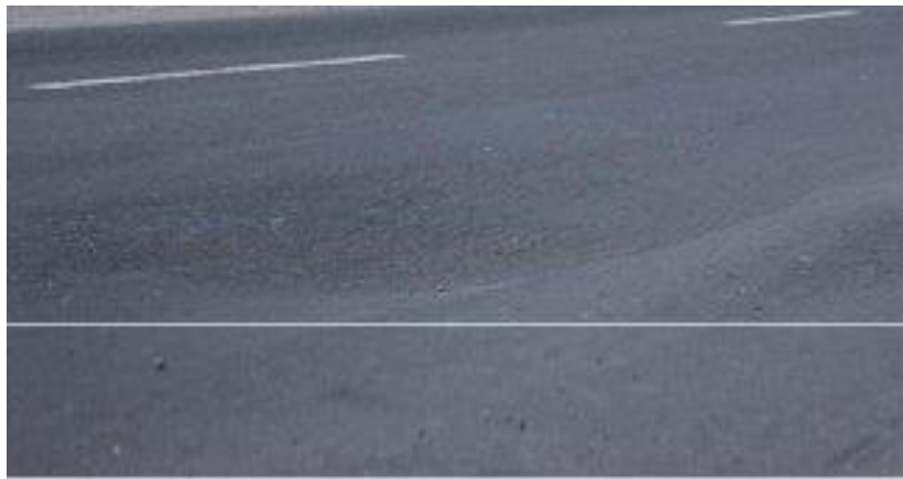
Gambar 2.13: Amblas ( Grade Depressions ) (SOP PUPR 2016).
