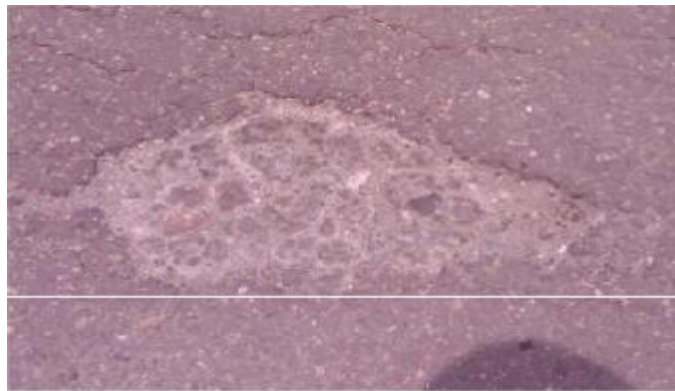
Gambar 2.18: Pengausan ( Polished Agregat ) (SOP PUPR 2016).
