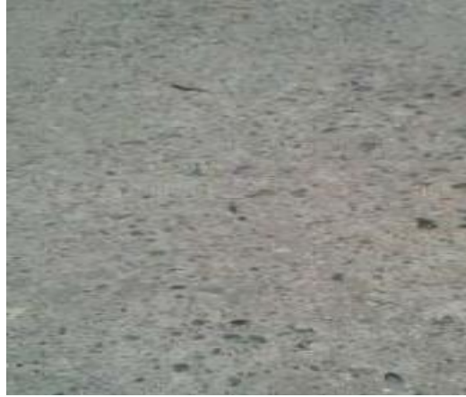
Gambar 3.7: Pelicinan ( polishing ) perkerasan kaku.
