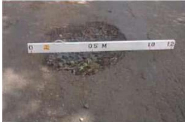
Gambar 2.4 Lubang (Pothole)
