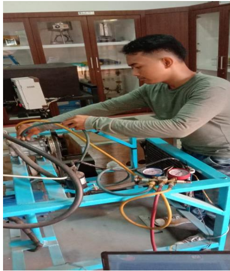
Gambar 4.2 Memasang manifold gauge
