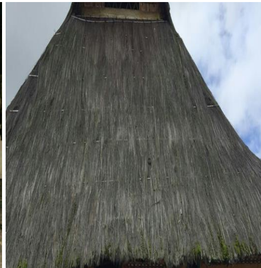
2.8 Tarum (Roof Made of ijuk)
