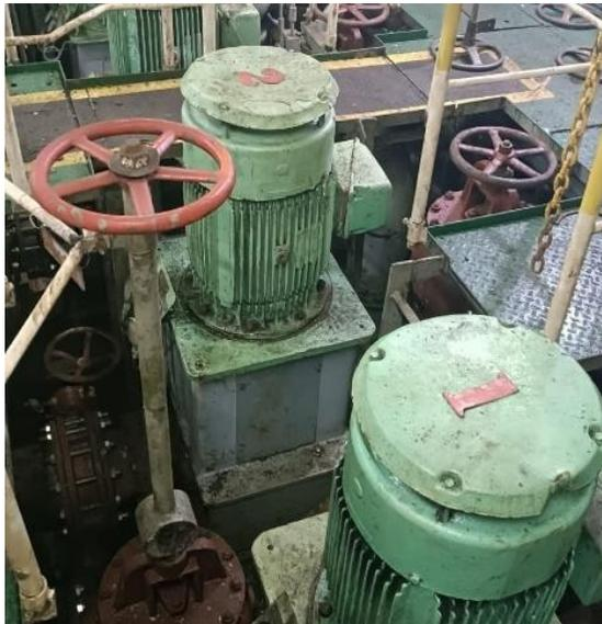
Gambar 4.3 Pompa Sistem Pendingin (Air Tawar)
