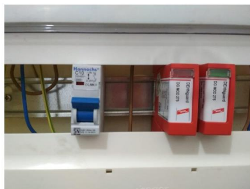
Arrester Accelerograph Red (Replace)
