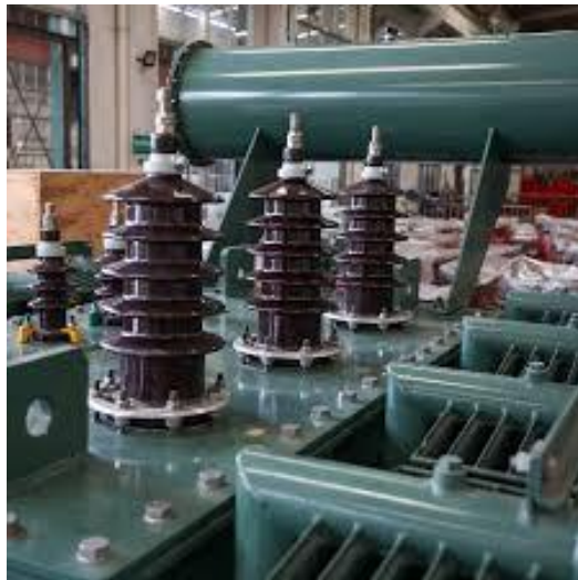
Gambar 2.6 Bushing Trafo
