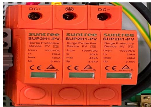
Gambar 2.4 Lightning Protection Systems
