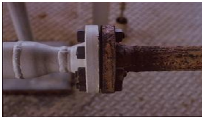
Gambar 2.5 Korosi Galvanik (Galvanic Corrosion)
