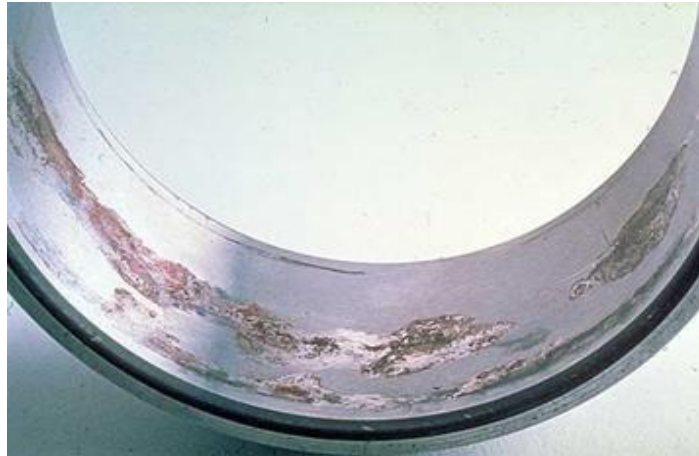
Gambar 2.9 Erosion –Corrosionand Fretting
