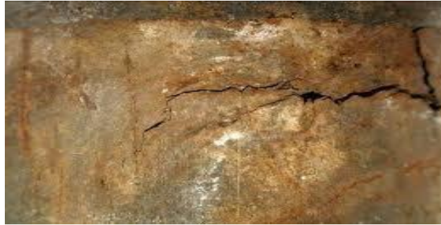
Gambar 2.8 Korosi Batas Butir (Intergramular Corrosion)
