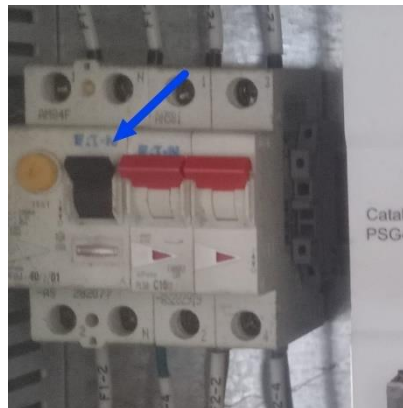
Gambar 2. 32 Elcb ( Earth leakage circuit breaker )
