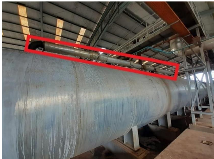
Gambar 2. 8 Pipa steam distributor
