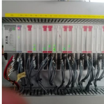
Gambar 2. 23 PLC ( programmable logic control )
