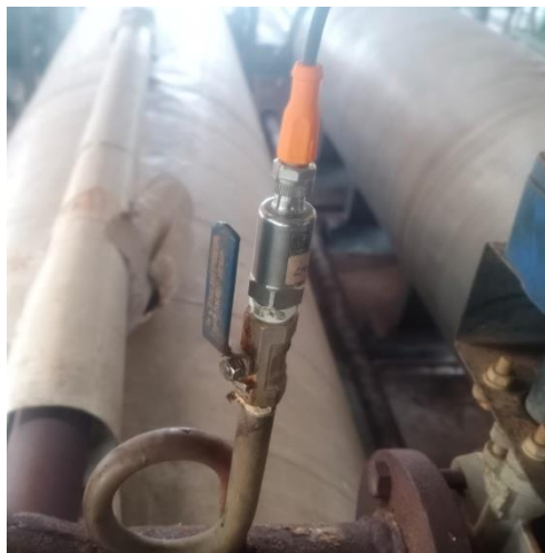
Gambar 2. 64 Sensor pressure transmitter
