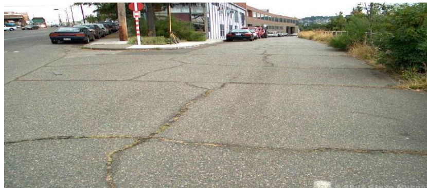
Gambar 2.12: retak sambung/ Joint Reflection Cracking (google)
