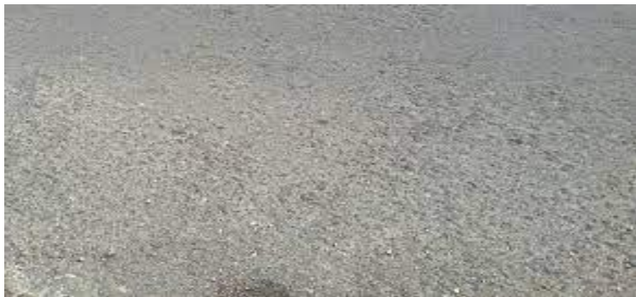
Gambar 2.16: Pengausan Agregat/ Polished Agregat (google)
