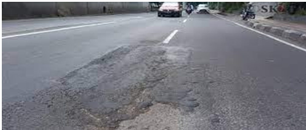
Gambar 2.15: tambalan/ Patching end Utiliti Cut Patching (google)
