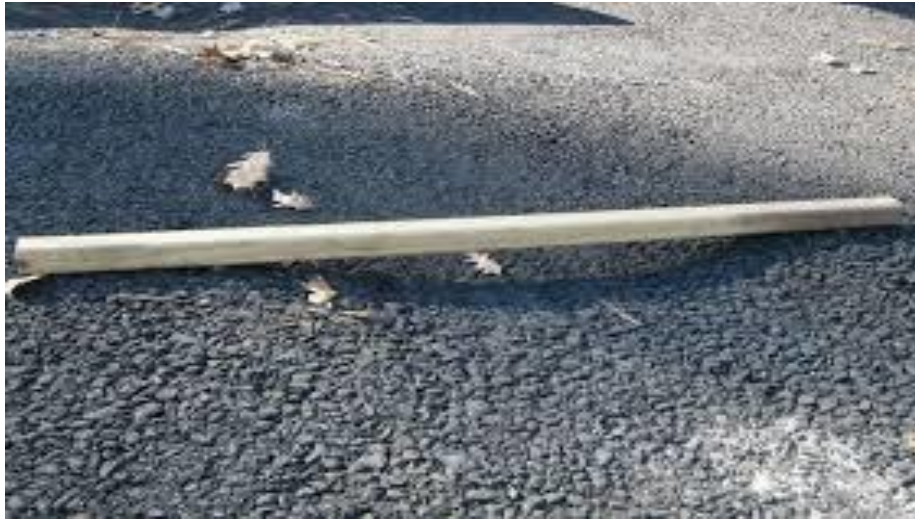
Gambar 2.23: pelepasan butiran/ Weathering and Revelling (google)
