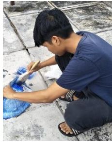
Gambar 4.4 Pelapisan Serat Fiber Glass
