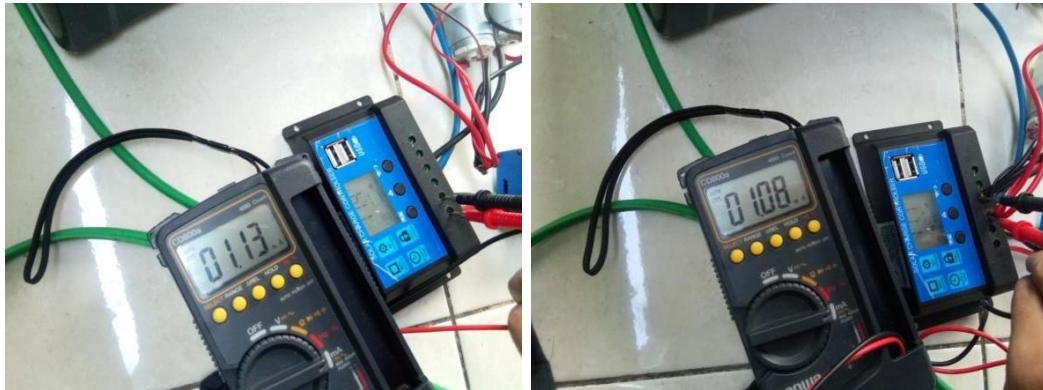
Gambar 4.18 V_{in} , I_{in} SCC & V_{out} , I_{out} SCC
