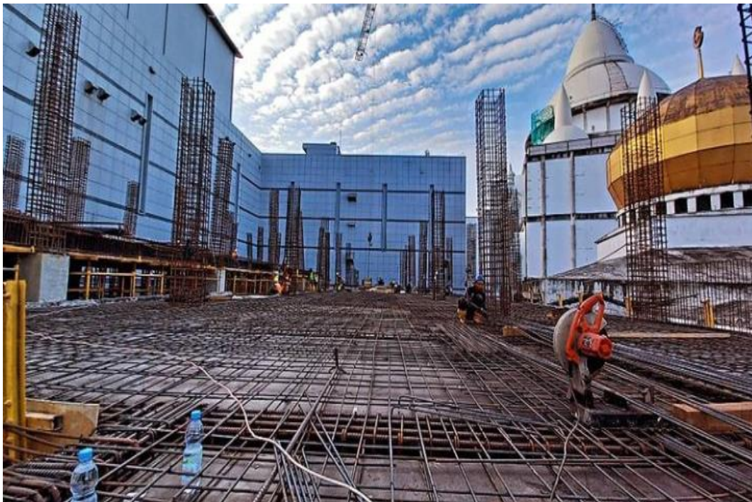
L2: Installasi Besi Lantai
