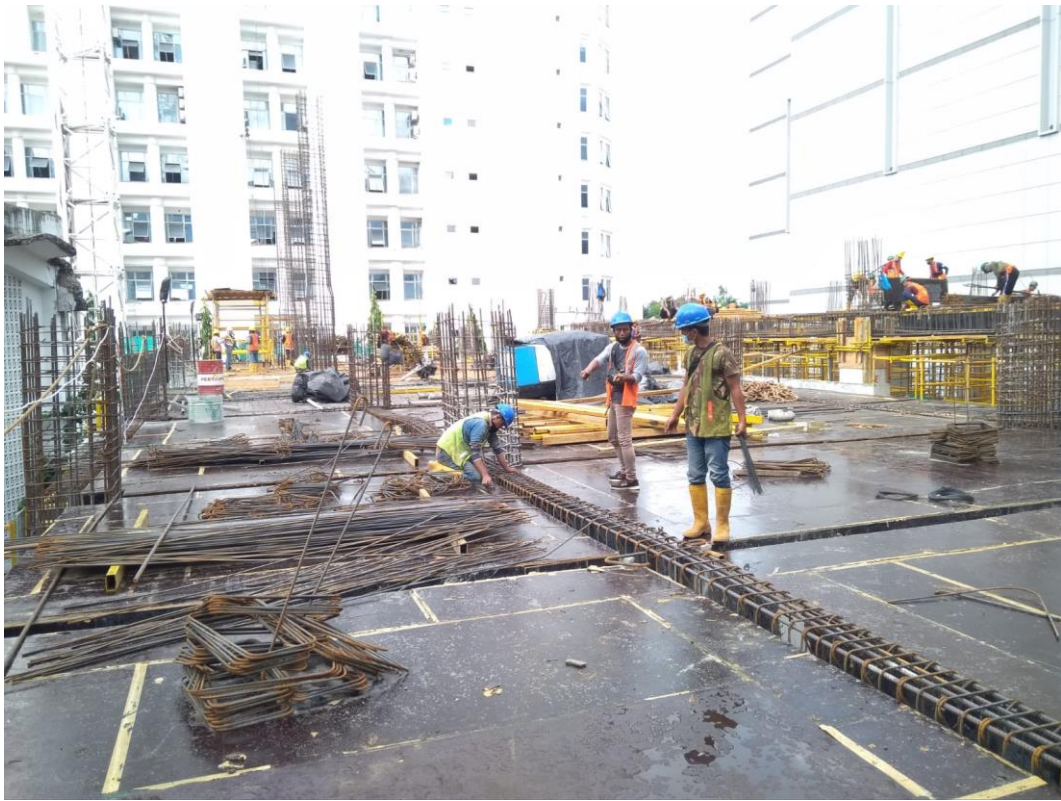
L1: Installasi Besi Balok
